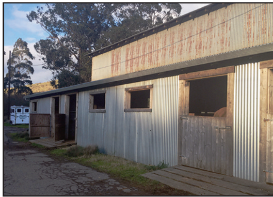
View of the dairy barn
